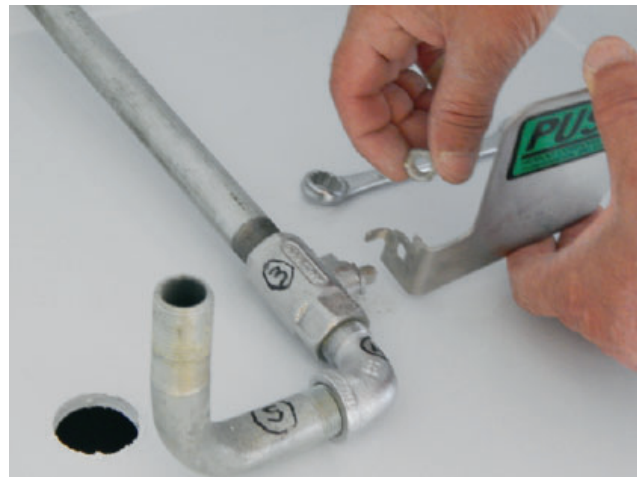
Install Push pull handle onto valve #3 using nut provided
